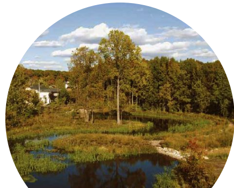
Trickling Filters and Vertical Treatment Wetland
