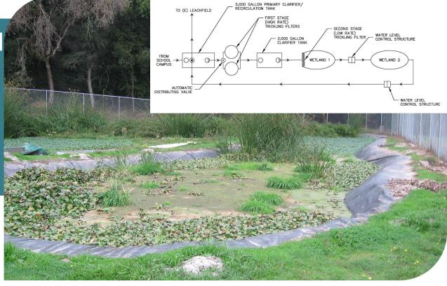
The system was installed in 2005. Regular maintenance activities include visual inspection and cleaning of biotube effluent pump vaults and pump systems. Other tasks include cleaning trickling filters monthly, and pumps the primary and secondary clarifiers annually.
