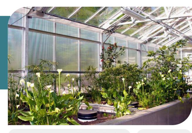
The Living Machine® system at Old Trail School in Ohio is an advanced wetland system, composed of primary settling, three different wetland processes (Horizontal Subsurface Flow, Tidal Flow and Vertical Flow), and UV disinfection which treat 5,000 gallons of wastewater per day.
