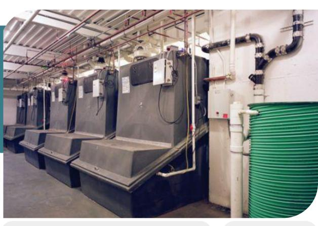
Completed in 2006, the Eco Restroom at the Bronx Zoo replaced a failing septic system. The system has an educational component, with signs which explain the composting toilet process to the public. The system was selected as an alternative to an expensive connection to the combined sewer system, or a new septic system, which was rejected due to pollution concerns. The greywater garden irrigates approximately 1,000 sq. ft.
