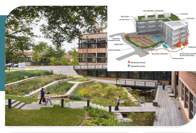
Onsite treatment of greywater and blackwater from a combined 72,000 sf existing and new buildings. Treatment process includes pretreatment tank to remove solids, subsurface flow wastewater wetlands, trickling filter, recirculating sand filter, and UV disinfection. Hydraulic residence time (HRT) in wetland is 3-5 days before entering storage tank in basement of building. When there is demand, water is then filtered and disinfected prior to reuse.
