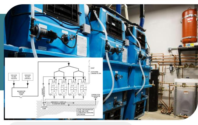
The building reduces water use by means of waterless urinals, composting toilets, and low flow fixtures, and harvests and stores rainwater on site. The composting toilet system (Phoenix) uses wall-mounted vacuum flush toilets (JETS) with a macerator pump which helps distributes material. The in-ground leachate tank is produced by Oldcastle. Operations staff adds wood chips and mixes bins weekly. System is oversized so they have only removed one batch of finished compost in the last three years.
