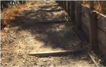
Pedestrian Paths, Stairs, & Retaining Wall
