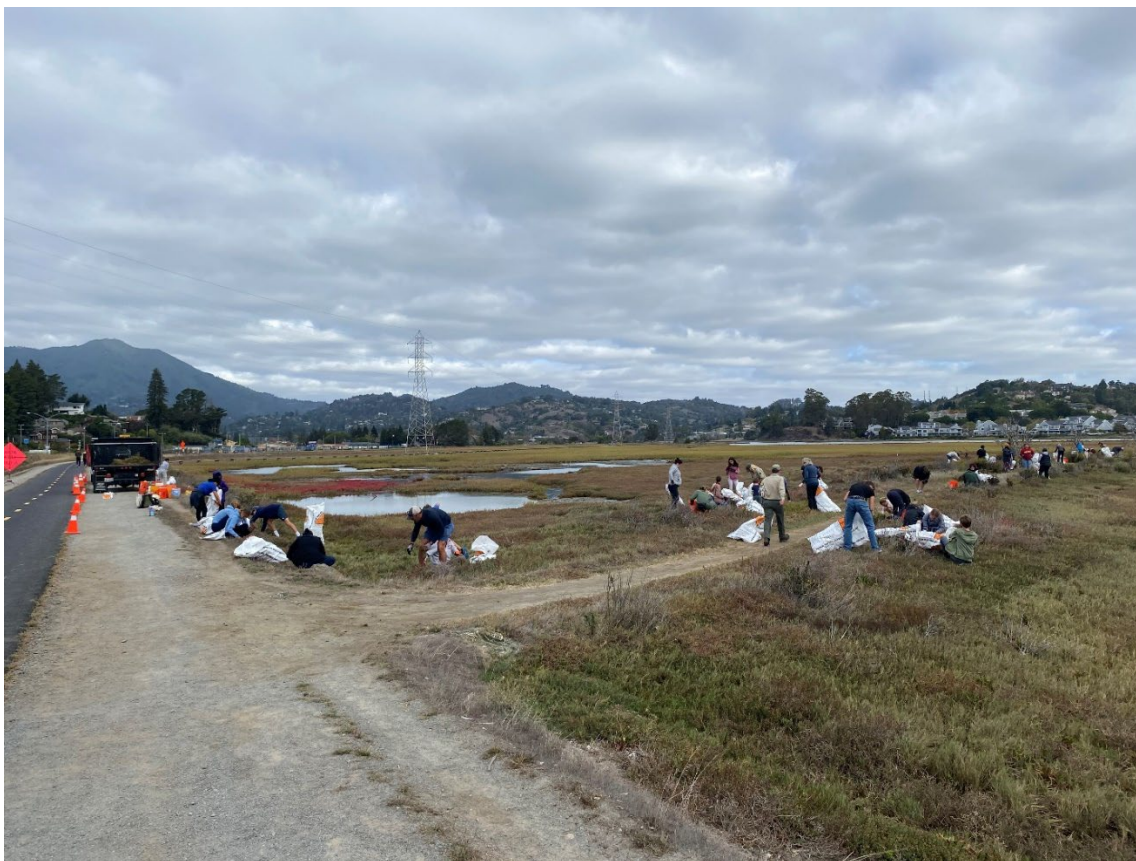
Above: Restoration work along the Mill Valley Multi-Use Pathway, October 2, 2022.
