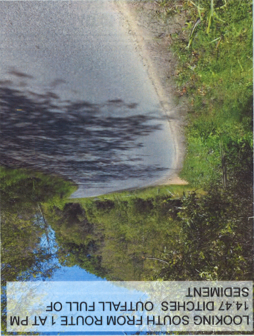
LOOKING SOUTH FROM ROUTE 1 AT PM 14.47 DITCHES AND CULVERT OUTFALL FULL OF SEDIMENT
